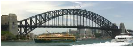
An Arch Bridge can be built using: wood, stone, steel or concrete
