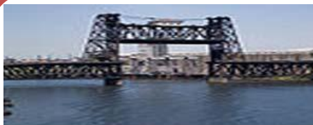
A Vertical Lift Bridge rises from the pillar supports to allow passage
