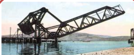
A Bascule Bridge is designed to lift vertically at one end at a pivot point to allow passage
